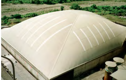
Purpose: Coal Storage Span: 60 m span irregular shape Industry: Cement Location: I-Lan, Taiwan
