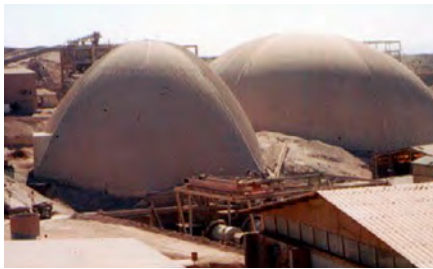
Purpose: Fine Materials Storage Span: 2 Freedom@s 60 m span Industry: Mining Location: Antofagasta, Chile
