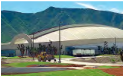
Purpose: Manufacturing Facility Span: Freedom® 224 m x 85 m Industry: Automotive Location: Monterrey Mexico
