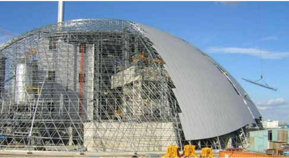
Geometrica's structural system permitted simultaneous construction of this waste-to-energy plant and the elegant dome enclosing it in Hampshire, U.K. Geometrica's modular technology allows construction from the perimeter up. English steel decking covers the dome, supporting the breather membrane and the external aluminum cladding.
